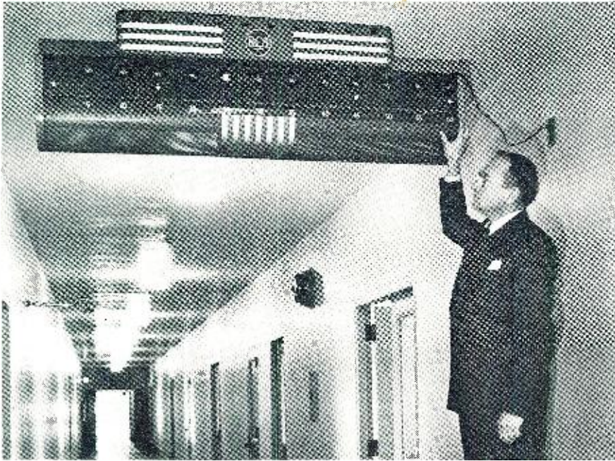
Novel electronic clock has more than 170 tubes that count 60-cycle pulses.
